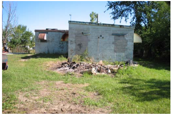
Photograph 1: View of the south (rear) side of the main building. Debris is present in the center of the old radar tower footings.
