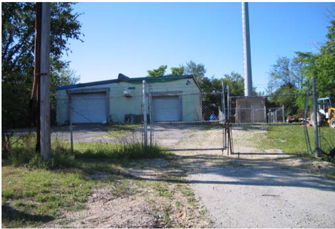
Photograph 1: View of the north side of the main building and the cellular phone tower in the southwest corner of the fenced portion of the property.
