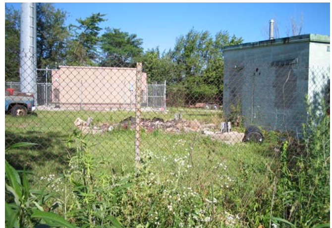
Photograph 4: View of the south side of the main building and east side of the cell tower building.
