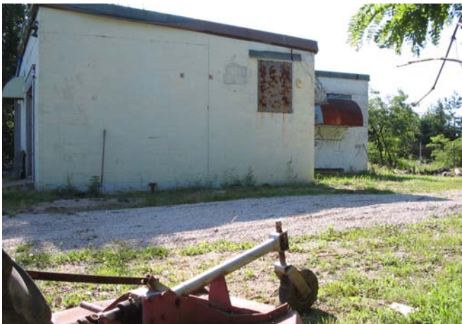
Photograph 3: View of the west side of the main building.
