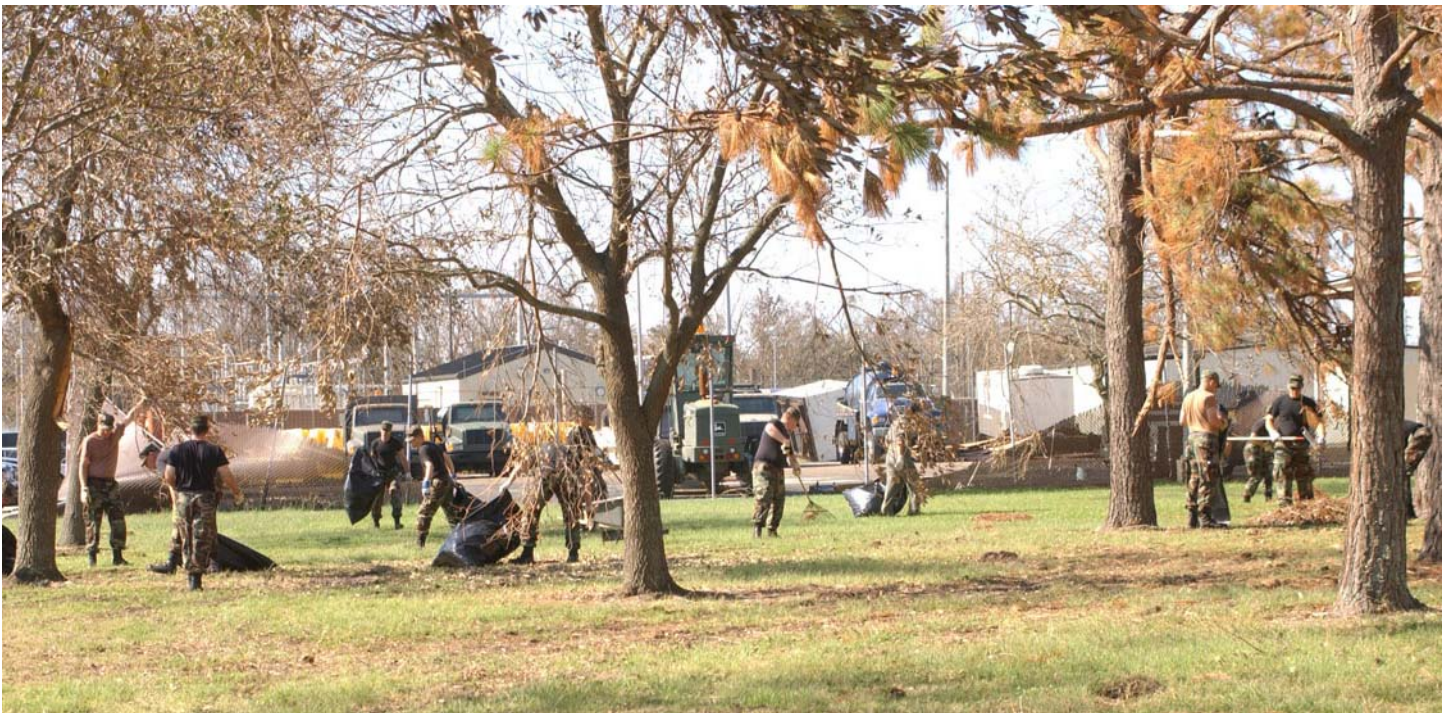
Keesler Airmen fan out to collect Hurricane Katrina debris here Thursday. After 823rd RED HORSE Squadron teams cut and removed the large portions of fallen trees, base detail members are working hard to improve the base's appearance. (Photo by MSgt. Dan Oberly)
