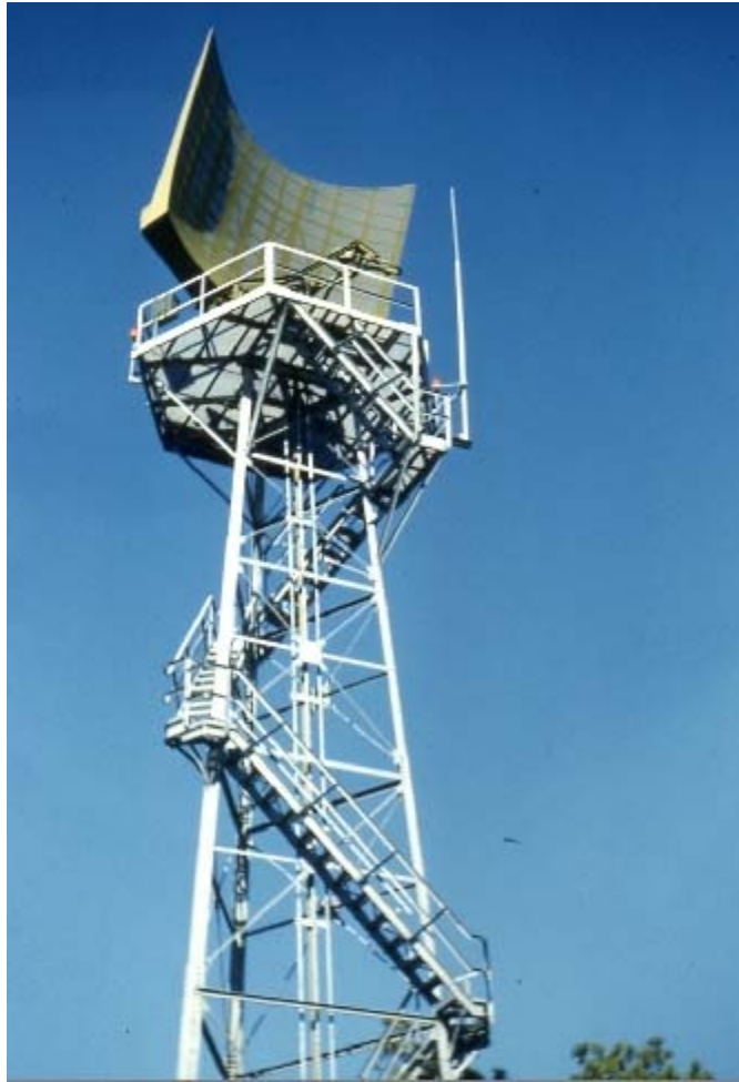
AN/FPS-14 Gap-Filler Radar (Myrtle Beach GFA, SC, circa 1962) (photo by Ken Dohrman)
