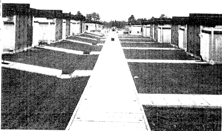
Figure 4. Covered Concrete Utilidors
