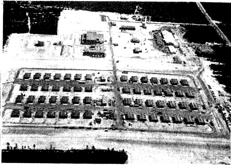
Figure 2. A 56-unit IM-99A Launcher Base under Construction
